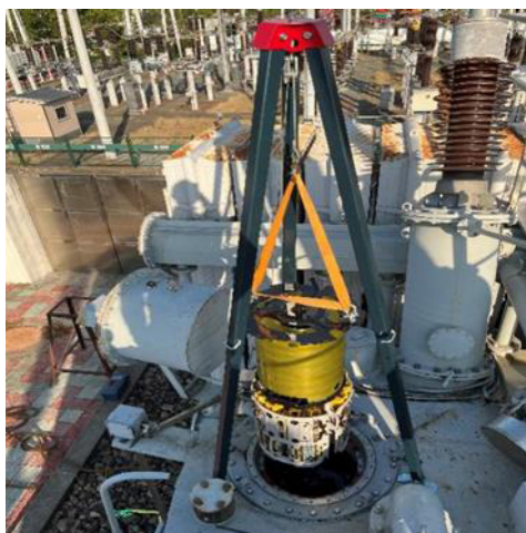
Fig.5 Triangular main transformer on-load tap changer hoisting equipment
