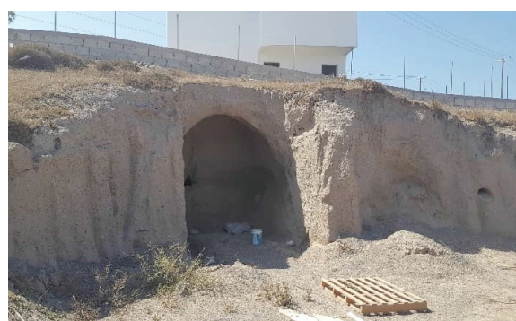
Fig. 1. The subsoil as seen in an open cut excavation in the area of the project.
