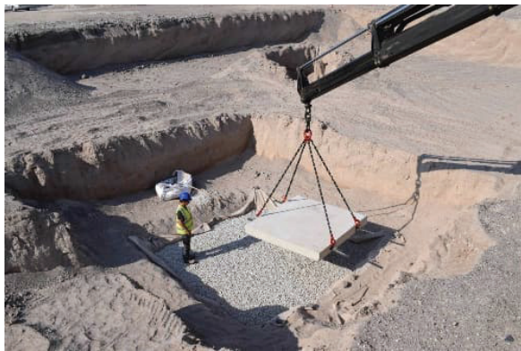
Fig. 5. Preparation for the load test.
