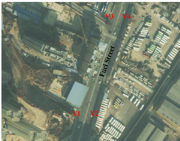
Fig. 1. Roadside monitoring system deployment.
