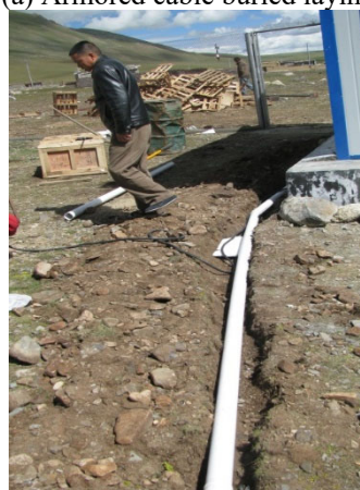
(b) PVC casing laying
