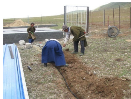
(a) Armored cable buried laying
