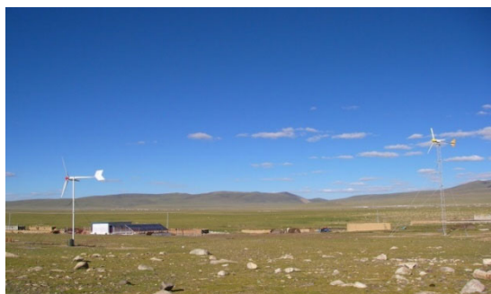
Fig.2 20kW wind solar complementary coupling power station after completion (left: 5kW fan, middle: 5kW photovoltaic, right: 10kW fan)
