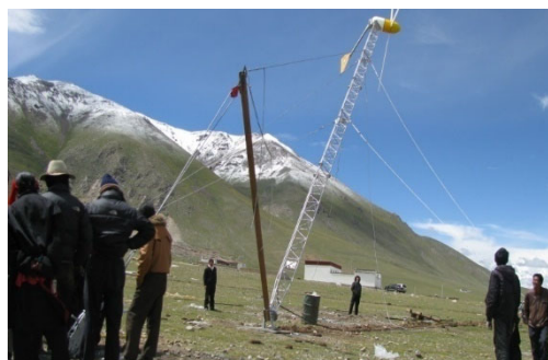
Fig.4 Fan installation site
