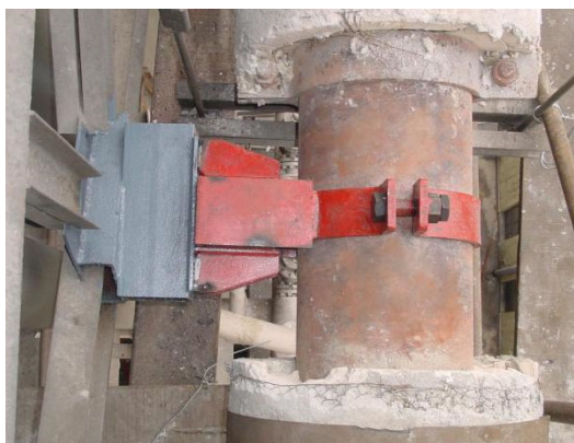
Fig. 3. Site installation drawing of No. 22 support and hanger limit.
