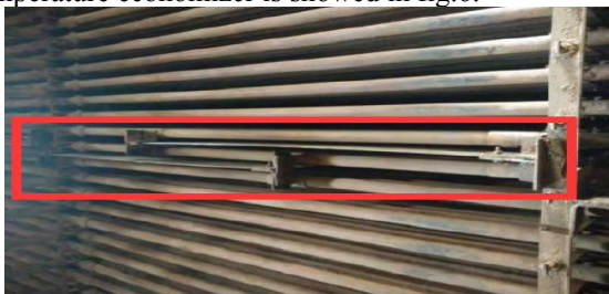
Fig.6. The clapboards' installation at the low temperature economizer on site.
