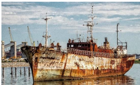
Fig. 2. Corrosion of vessel components
