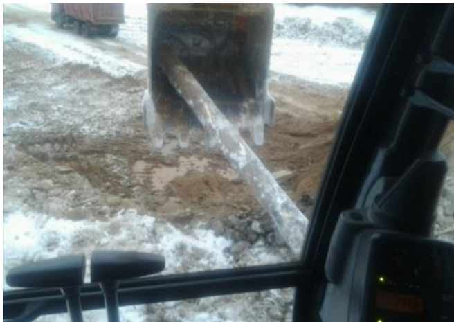
Fig. 3. Manual cleaning of the bucket with the help of improvised devices.
