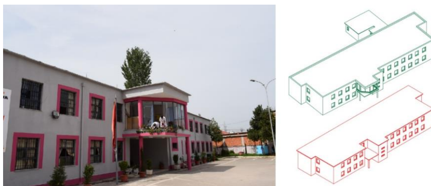
Fig. 2. Main facade of the school and comparison current situation (green) and original design (red) - (source: the authors)
