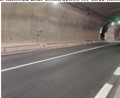
Fig. 2. Effect of one month after construction.
