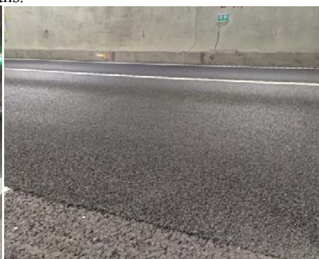
Fig. 3. Effect of three months after construction.
