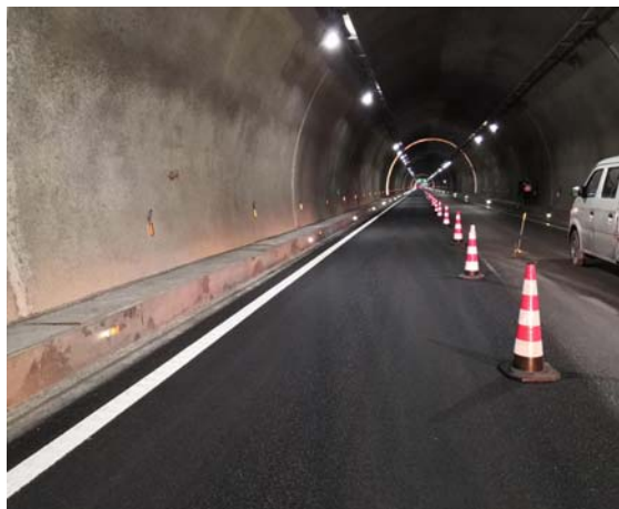
Fig. 1. Effect after construction completion.
