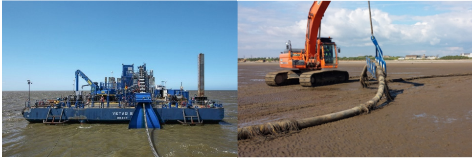
Fig. 10 CLV VETAG 8 and crawler excavator into intertidal zone [5]
