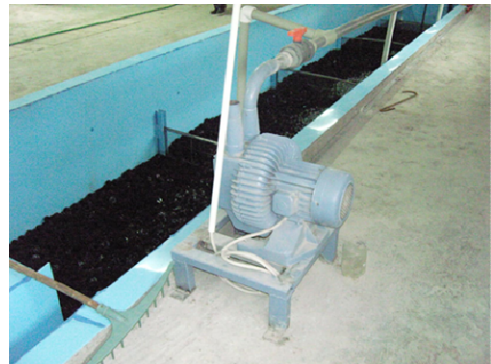
Fig.3 Aeration system of the biological filter
