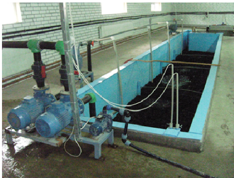
Fig.2 Biological filter with ball
