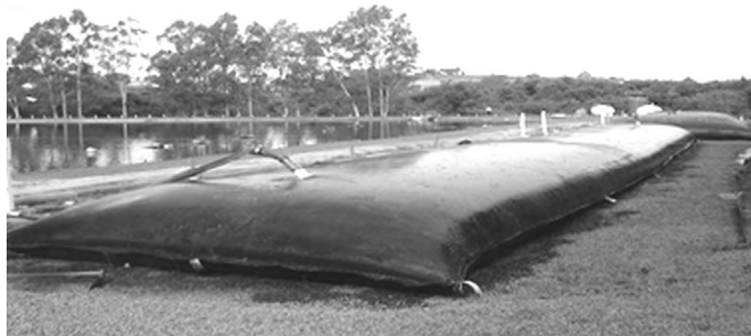
Fig. 2. Geotube in working condition.
