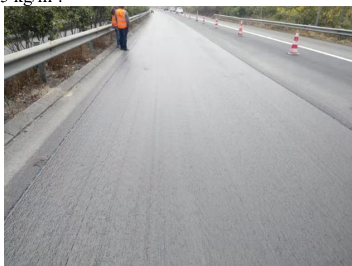
Figure 1 Existing Pavement Treatment
