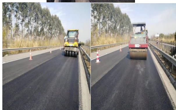
Figure 3 Combined Steel-Rubber-Steel Rolling Compaction Process
