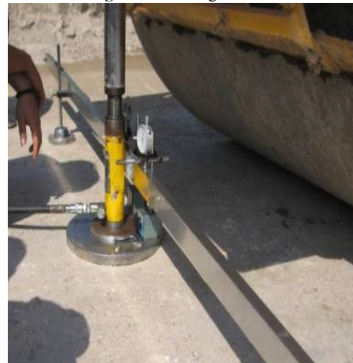
Figure 2. K30 plate load test
