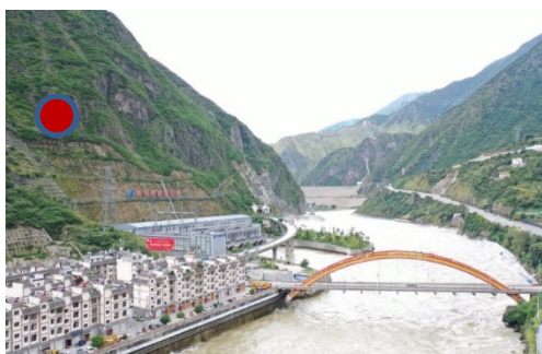
Figure 2. Entrance of Baolingshan Tunnel
