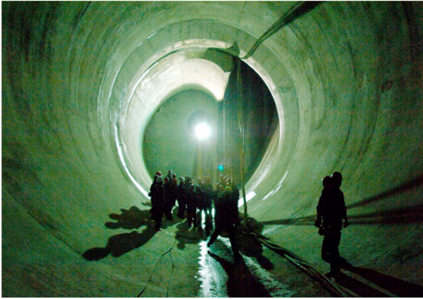
Fig. 2. The Generator of Flood Discharge Tunnel with level swirling flow
