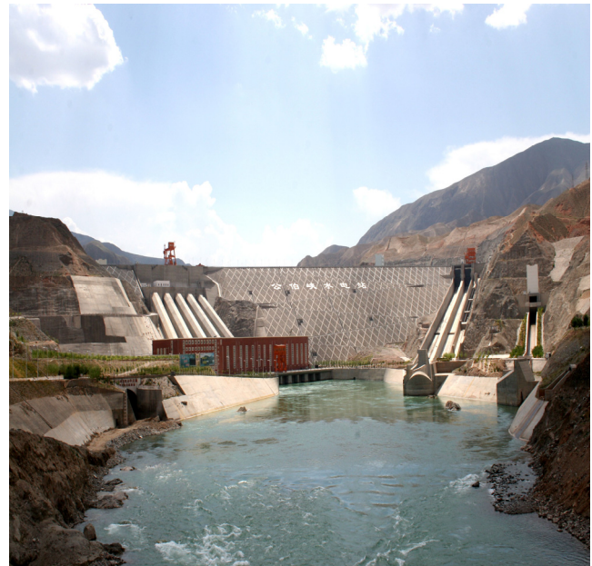
Fig. 1. Panorama of Gongboxia Hydropower Station
