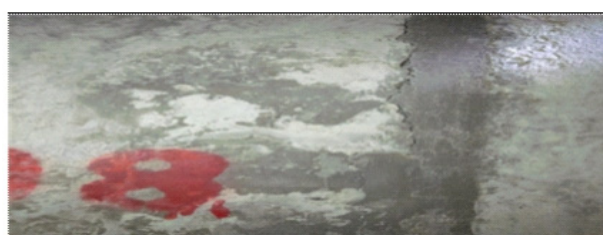
7#Yinyangxia culvert, Stake 86+469.08
