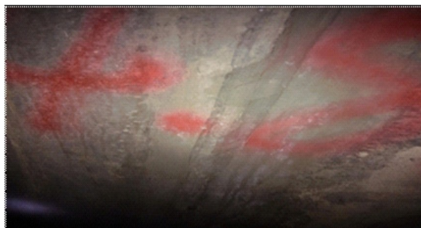
12 # Wulongchuan culvert, Stake 90+495.16
