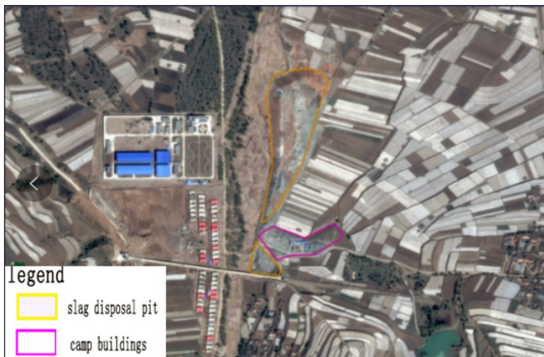
Slag dump and construction site at 10# tunnel entrance of main canal (image in 2014)
