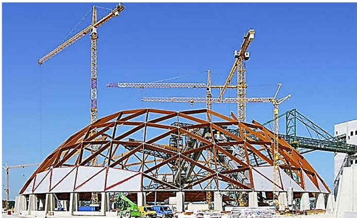
Fig. 3. Installation of the geodesic dome structure.
