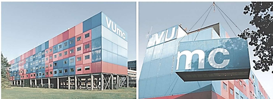
Fig. 10. Design and assembly of modular containers [19].
