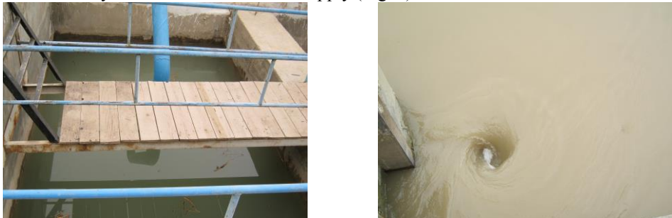
Fig. 2. Studies of the flow supply of the PS "Babotag" in the conditions of funnel formation
