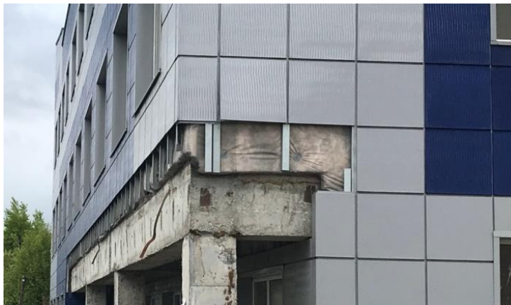
Fig. 3. Contamination of the moisture-windproof membrane during operation
