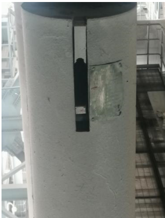
Figure 1 Indicating an abnormal state of the spring hanger
