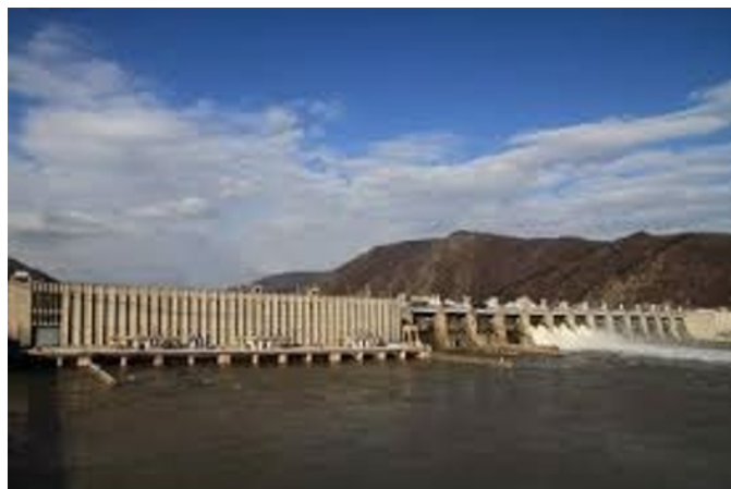
Fig. 1. Djerdap (Iron Gate) hydro plant Source: http://www.tos.org.rs/node/990
