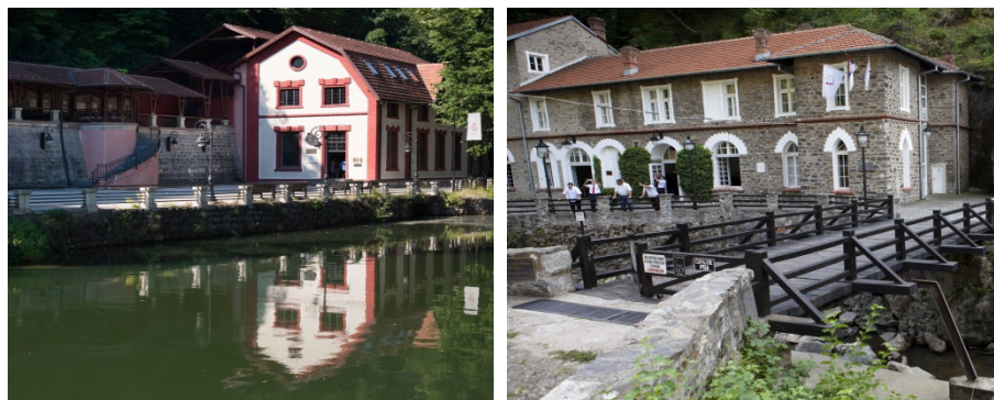
Fig. 2. Hydro plant Pod Gradom (left) and Vucje (right)
