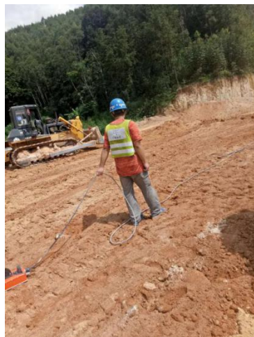
Fig.3 On-site inspection photos
