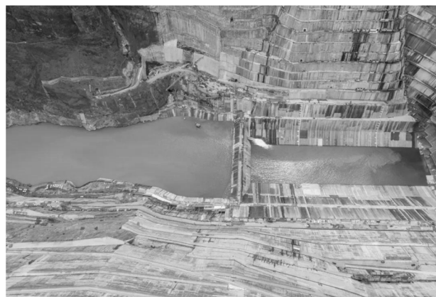
Fig.4 Effect diagram of the first water filling process in the cushion pool of the project
