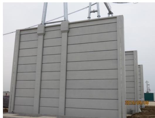
Fig. 13. Photo of Fabricated firewall completed product
