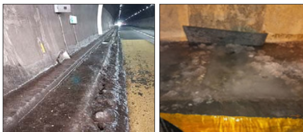
Fig. 3. Freezing of Tunnel Pipe Trenches and Longitudinal Blind Drain Manhole.
