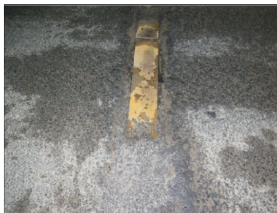
Fig. 10. Design of Pavement Slotting and Drainage.
