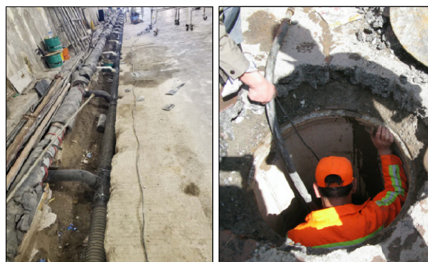
Fig. 8. Dredging of Roadside and Central Ditches.
