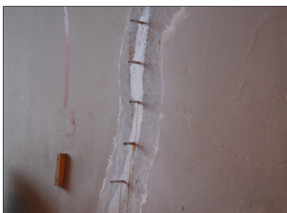
Fig. 6. Glue Injection and Sealing of Cracks.
