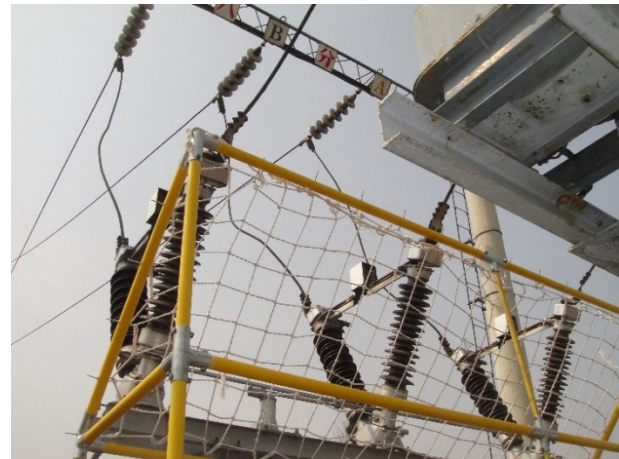
Fig. 6. Insulation protection frame field application effect picture
