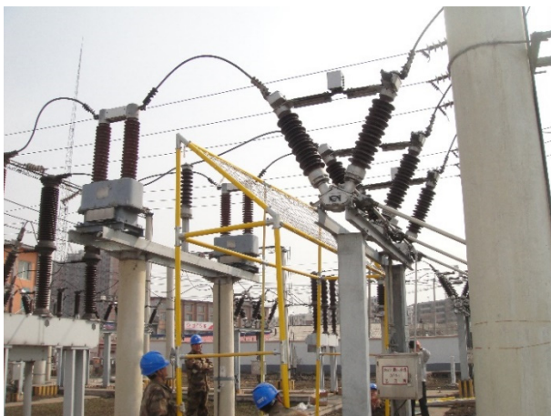
Fig. 5. Insulation protection frame operation site movement picture
