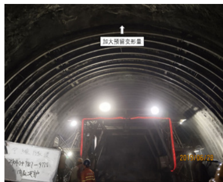
Fig. 9 Increasing Reserved Deformation of S3 Support
