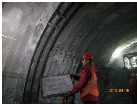
Fig. 6. Inner Primary Support of S1 Support Completed
