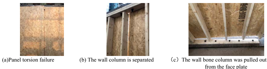
Fig2. Shear wall failure mode
