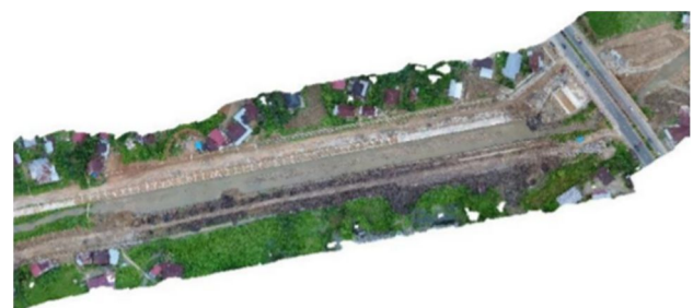
Fig. 2. Condition of Batang Maransi River.
