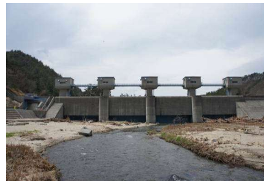
Fig. 16 Fudai water gate (downstream side)
