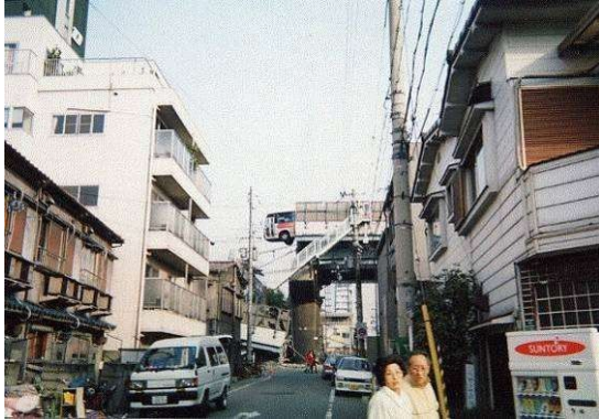
Fig. 1. A bus hangs over the edge of the collapsed highway
