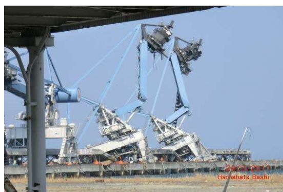
Fig. 13. Buckled crane arm (Soma)
