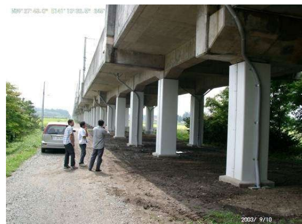
Fig. 22. Strengthened viaduct columns after 2003 Sanriku-minami-earthquake
