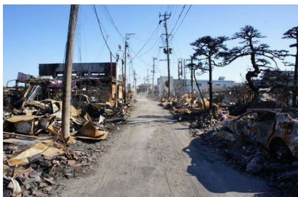
Fig. 10. Damage caused by fire after (Kita-ibaragi)
