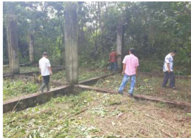
Fig. 1. Existing Building Condition
