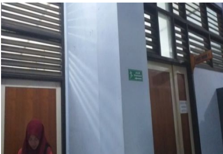
Fig. 7. For an example of a misplaced and misused evacuation symbol on Building A, here a ladder symbol was used on a straight path.
