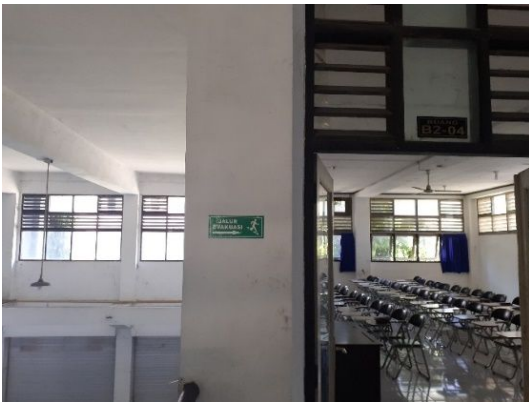
Fig. 12. Example of a misplaced evacuation symbol on Building B, which is quite impossible to be seen by the people who come out from the classroom.
