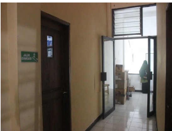
Fig. 14. A misplaced evacuation symbol on Building C1 might be misunderstood there is a staircase behind the door.
