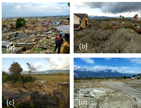
Fig. 1. Flow liquefaction phenomena in (a) Balaroa, (b) Petobo, (c) Ojo Oge and (d) South Sibalaya.
