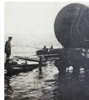
Figure 8. Delivery of tanks in the Baku port
