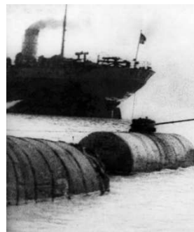
Figure 7. Fastening of tanks to the towing rope
