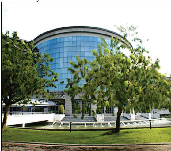
Fig.1. UNITEN administration building.
