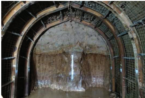
Fig. 4. Appearance of lapilli tuff on the inlet tunnel face
