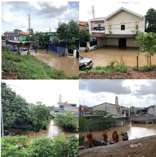
Fig 9. Flood condition in RW. 04, Cipinang Melayu.
