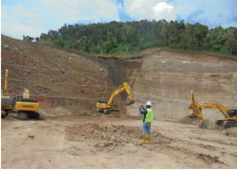
Fig. 4. Moderately to highly weathered andesite.
