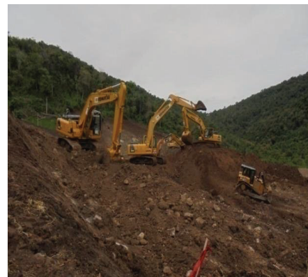
Fig. 3. Colluvium consists of black clay and 2 – 10 cm andesite fragments.
