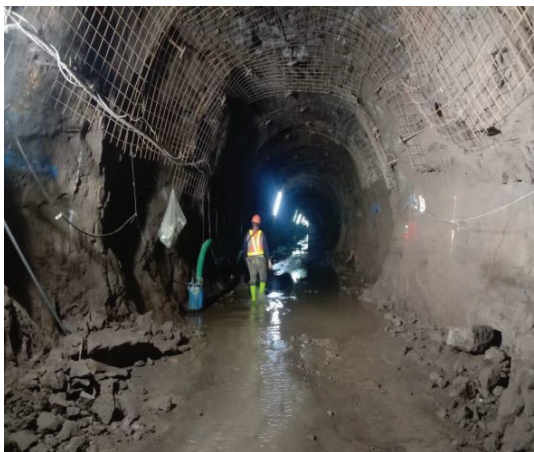
Fig. 11. Rock bolt, wire mesh, and shotcrete installations.
