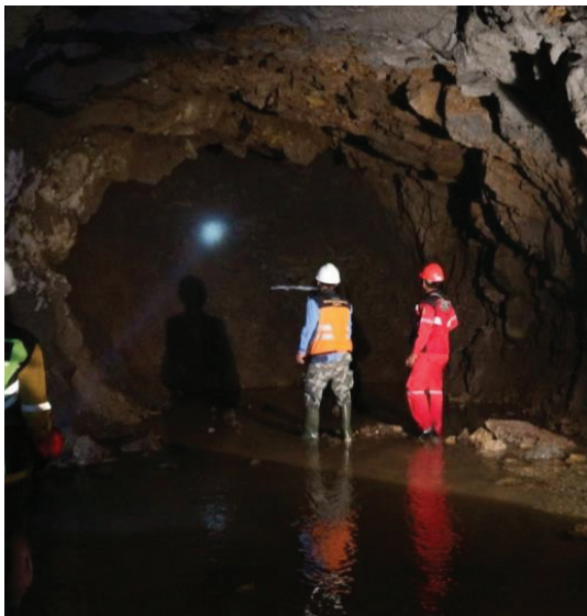
Fig. 10. Typical rock mass condition after blasting.
