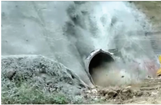
Fig. 9c. Tunnel excavation: Blasting.
