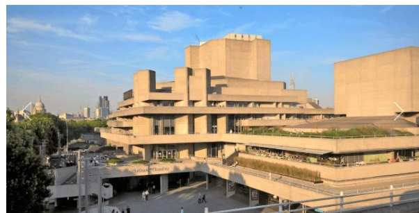
Fig. 1. Sir Denys Lasdun's Grade II* National Theatre. Photo by Mark Hammond (via Enrich the List)
