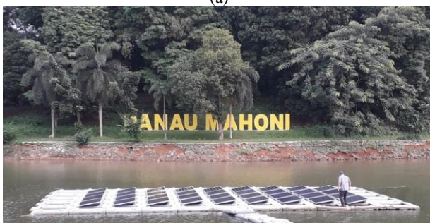
Fig. 1. (a) Rooftop Solar PV System and (b) Floating Solar PV System
