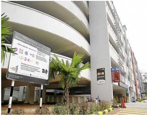
Fig. 2. Six-story intercept parking lot in Malaysia.
