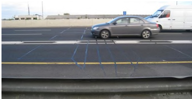
Fig. 2. Induction loop detectors–transportation.
