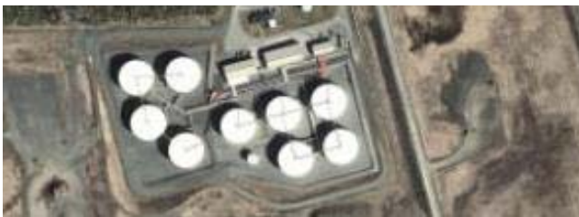
Fig. 2. Oil storage tank image example
