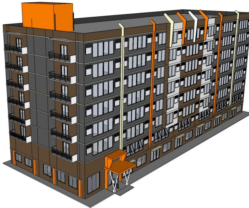
Fig. 1. Overview of case study building.
