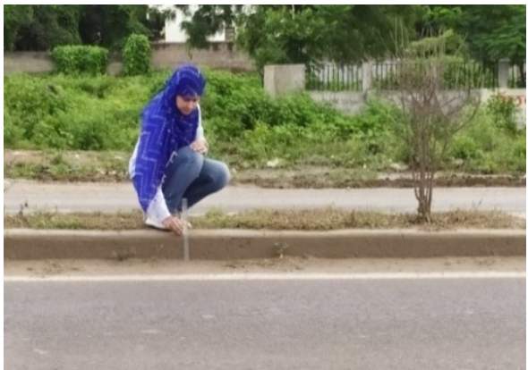
Fig.10 Insufficient Median Height
