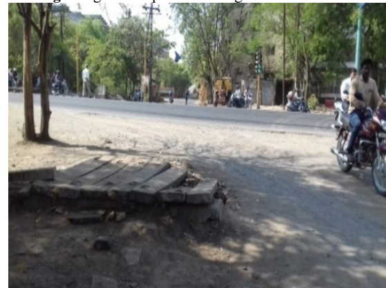
Fig. 5 Open Gutter on road side
