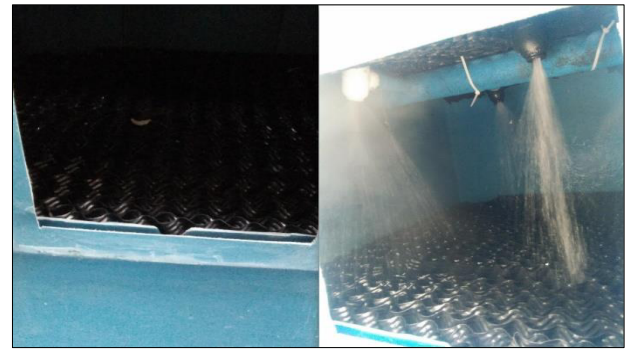
Fig. 5. Fills and drift eliminator
