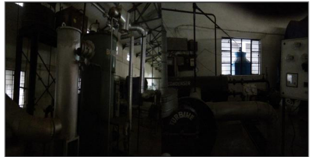
Fig. 2. Mini-steam power plant
